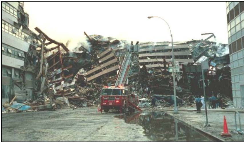
Figure A-6. Debris pile from collapse of WTC 7 onto the Con Edison substation, viewed looking south from Greenwich Street, date undetermined.
