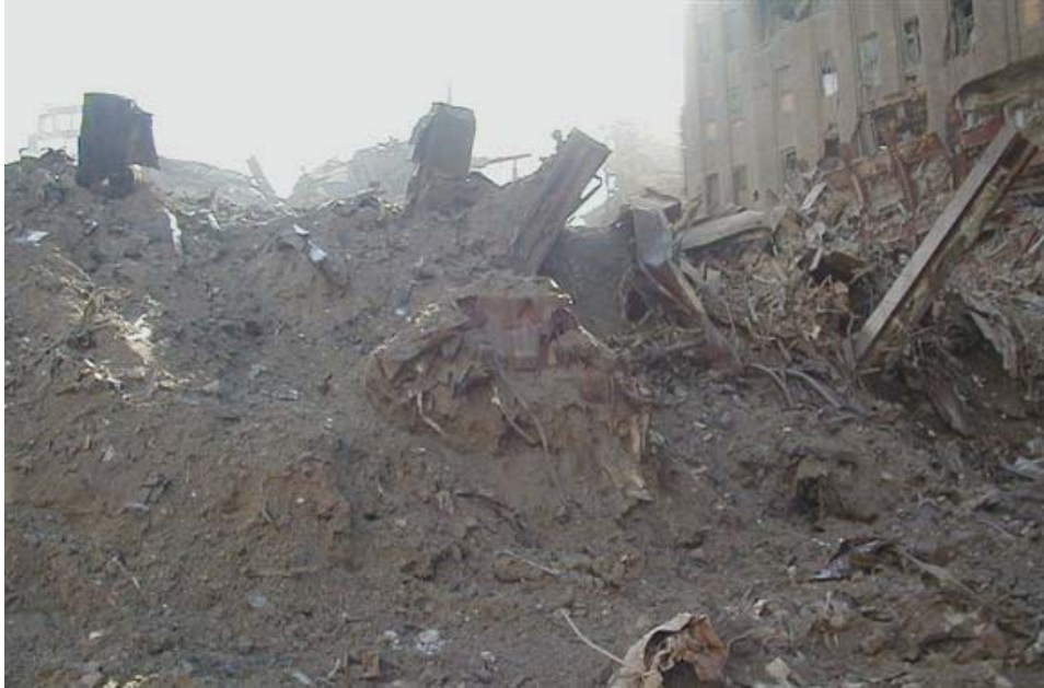
Figure A-9. Con Edison transformer #7 (or #5) uncovered from debris pile of WTC 7; photo taken mid-October, 2001.
