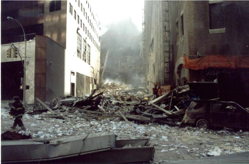
Figure A-4. Northwest corner of the Con Edison substation (building on left), showing light damage from WTC 1 debris. (Photo taken sometime in the afternoon on Sept. 11, 2001.)
