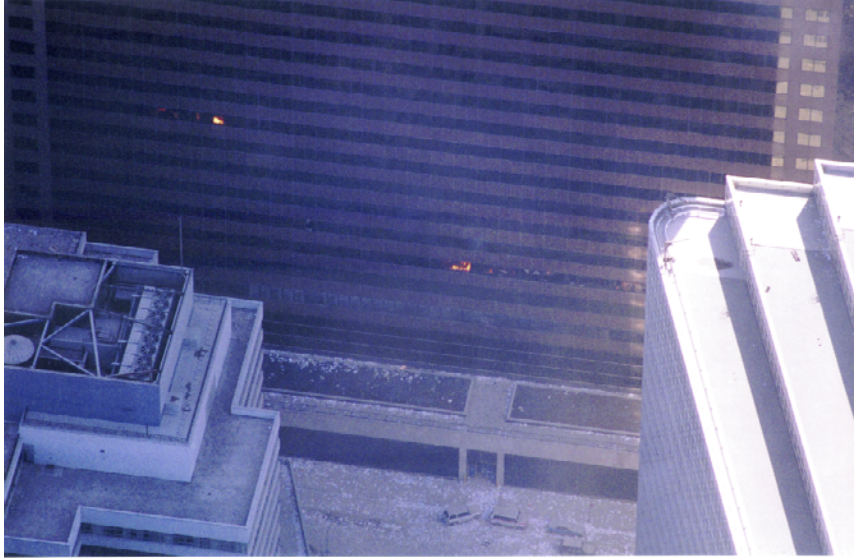
Figure A-5. Aerial view of the middle of the north side of the Con Edison substation, taken sometime between 1 p.m. and 3 p.m. on September 11, 2001.
