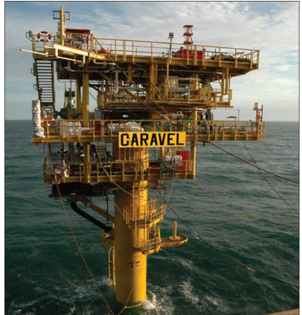
The joint-venturer-operated Caravel field in the U.K. North Sea is being developed with a monotower design.
