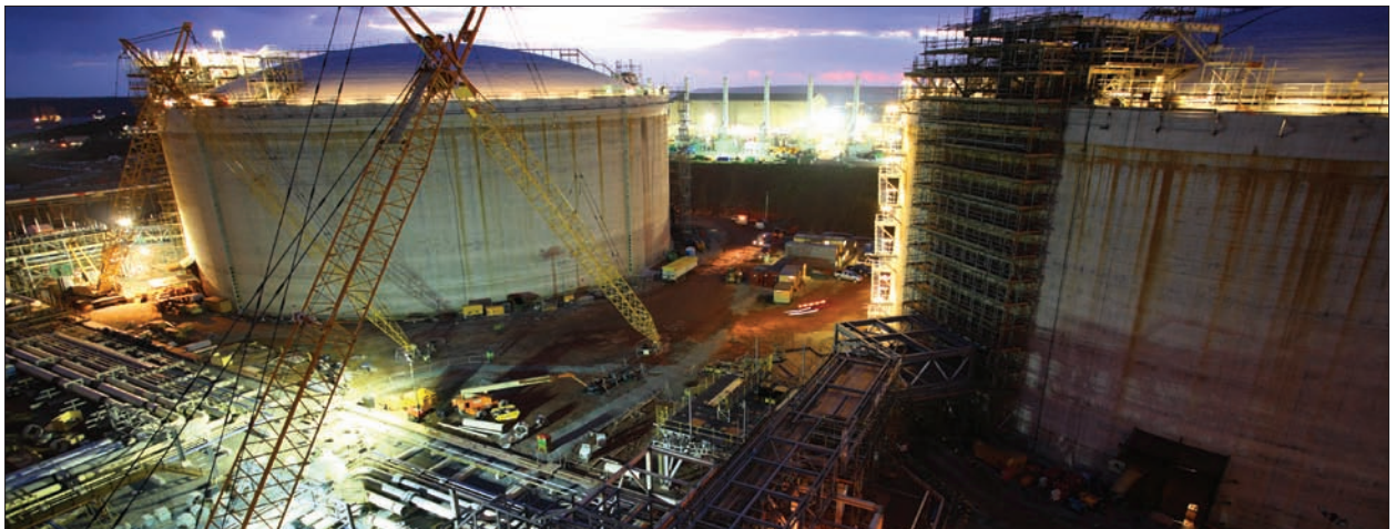
Construction progresses on the South Hook LNG regasification terminal in Milford Haven, Wales.
