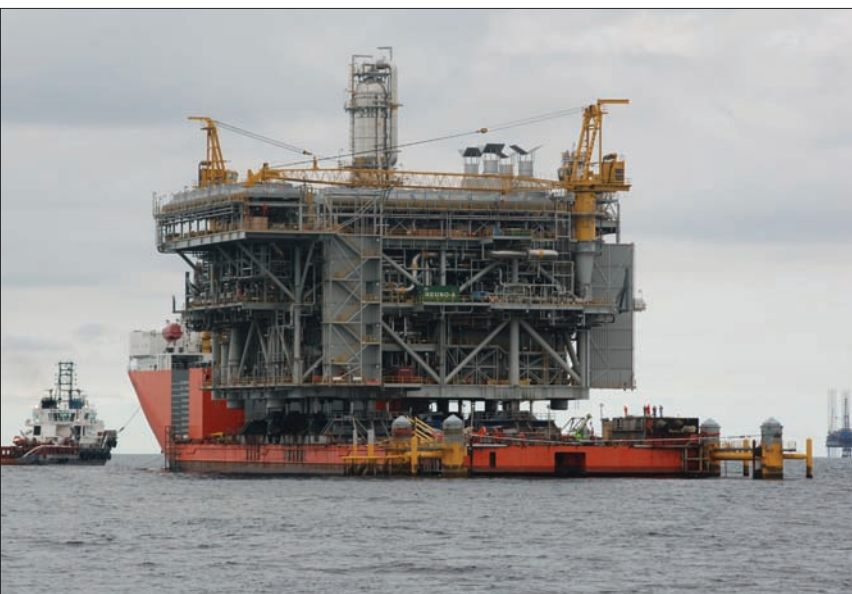
New production facilities for the East Area NGL II project offshore Nigeria were installed in 2007.
