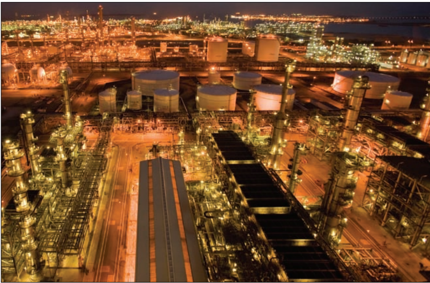
The Singapore Chemical Plant is fully integrated with ExxonMobil's largest refinery. The Singapore complex is one of the largest integrated manufacturing sites in the world.
