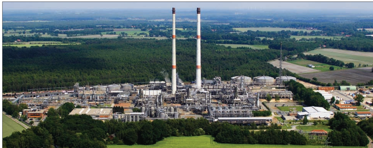
The Grossenkneten plant (ExxonMobil interest, 67 percent) started up in 1972. Sulfur is removed using three processing trains to improve the quality of the sales gas.
