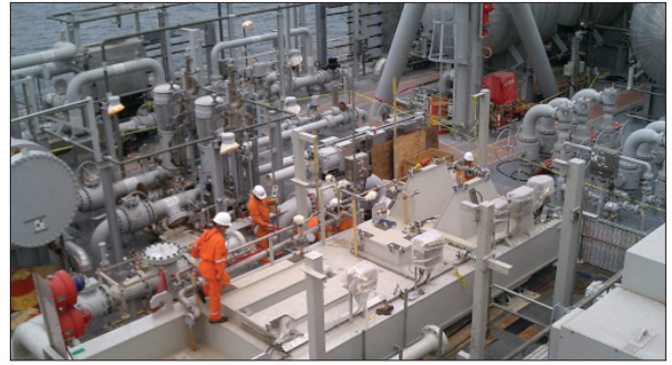
The Marimba North project, a subsea development offshore Angola that started up in 2007, utilizes facilities on the Kizomba A FPSO, shown here.
